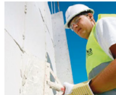
G. A spack knife for removing excess mortar.
