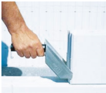
F. Silka thin bed mortar scoop, designed for the thickness of the elements used, which evenly applies the thin joint mortar to the vertical joints of the elements.
