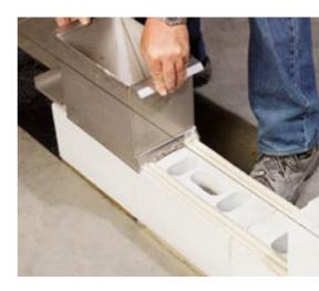
Specially designed thin joint mortar applicators and scoops are available for each wall thickness
