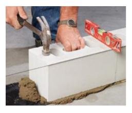
The first course of Silka CS blocks, called the 'kicker course', is constructed on a traditional mortar bed to ensure it is completely level. In doing so, irregularities in the floor can be corrected.
