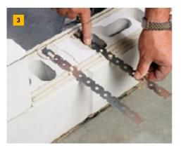
With the cavity wall anchors and the matching 'lip-clips', you can perfectly place the insulation against the wall.
